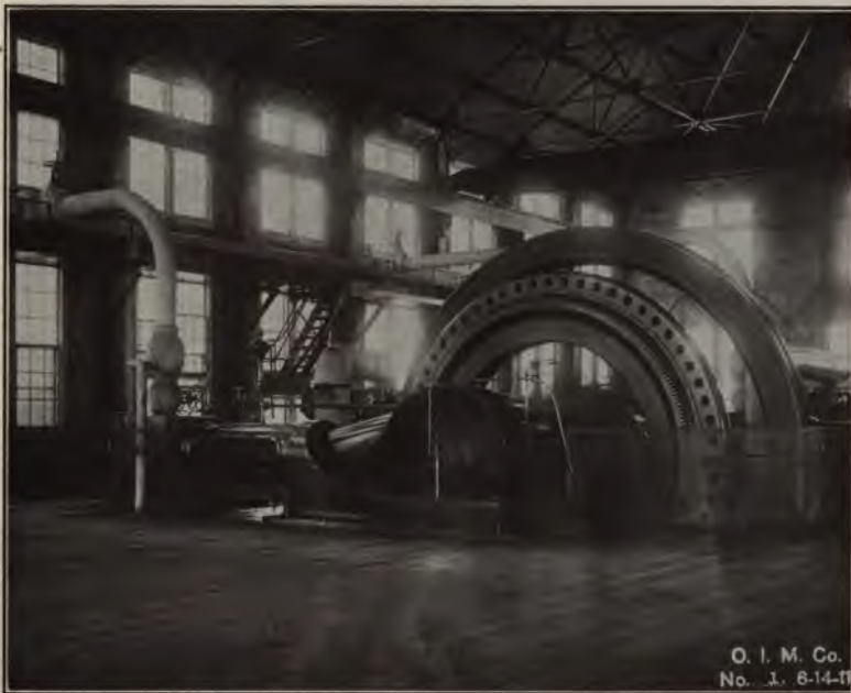
No. 1—Trout Lake Power Plant, Coleraine, Minn.
